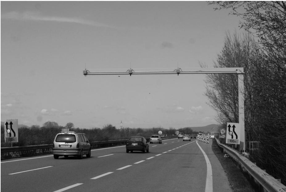
Figure 3.3 DSRC charge point (LKW Austria). (Courtesy of Kapsch TrafficCom AG.)
